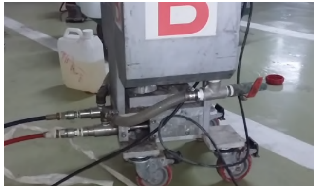
(11) Turn the power switch on for running machine, and inject the acrylic resin into every holes.
