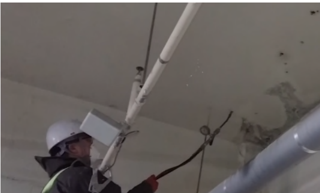
(10) Connect the acryl gun with installed packers.
