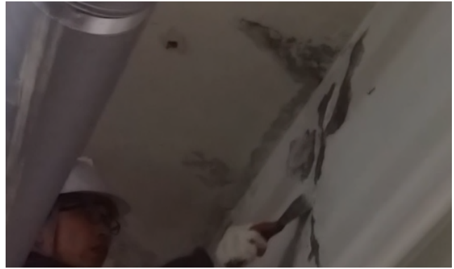
(13) Clean the holes/crack areas, and coat the sealing material.
