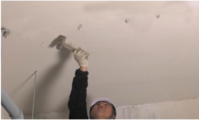
(12) After finishing injection, remove packers using a hammer.
